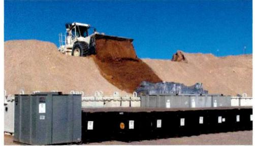
These containers hold the remnants of gloveboxes used in processing radioactive materials. Low-level and some mixed low-level waste is permanently disposed of onsite.
