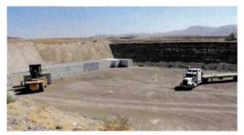
This is a typical disposal cell for low-level waste.
